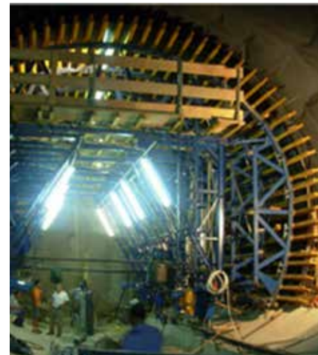
Custom traveling arch shaped formwork solution.
