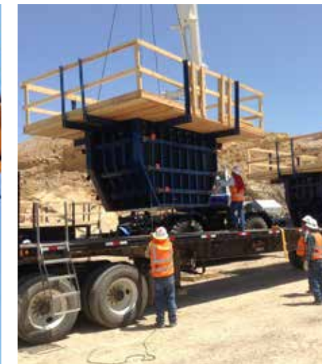
Pier Caps assembled off site and shipped to the project site.
