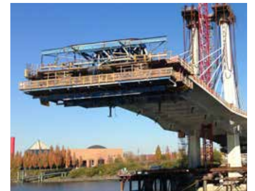
Custom, cantilever formwork & traveler system.
