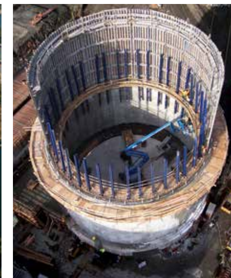
Radius form used in deep water diversion structure.
