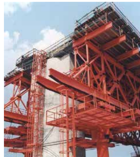
Fully automatic, custom steel launching system, used in bridge construction.
