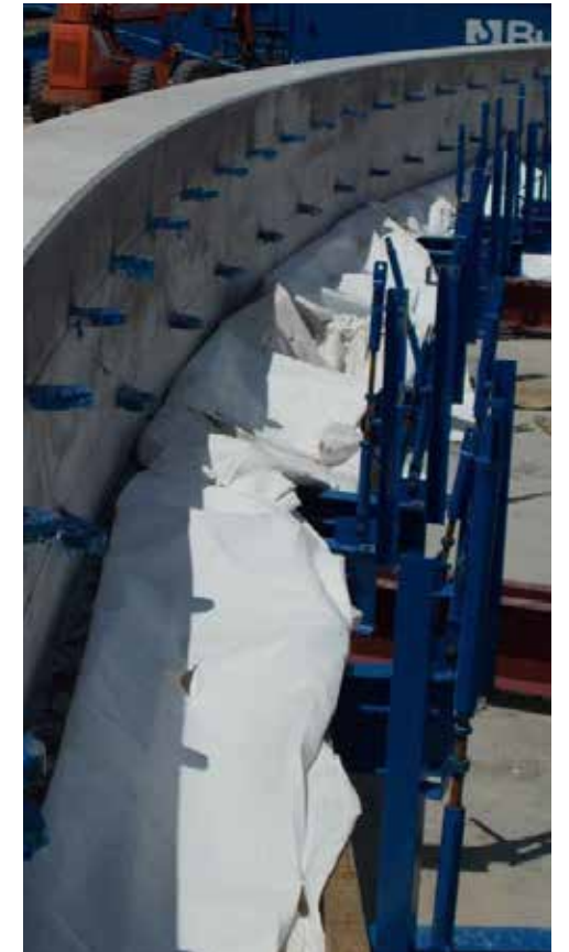
Custom steel pre-cast arch forms.
