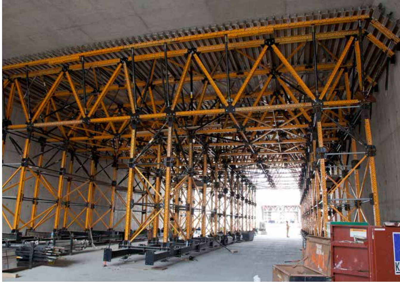
Rolling Track system utilizes standard equipment with minimal custom steel to deliver an extremely flexible and cost effective solution.
